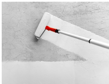
Fig. 3.7 Photo fragment of the method of applying the primer with a roller
