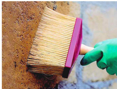
Fig. 3.6 Photo fragment of the method of applying the primer with a brush
